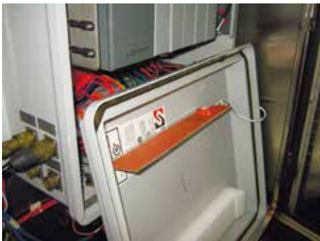
Automatic electric heater for computer System in the control console
