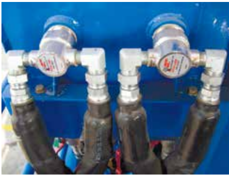
Hydraulic and lube fluid warmer
